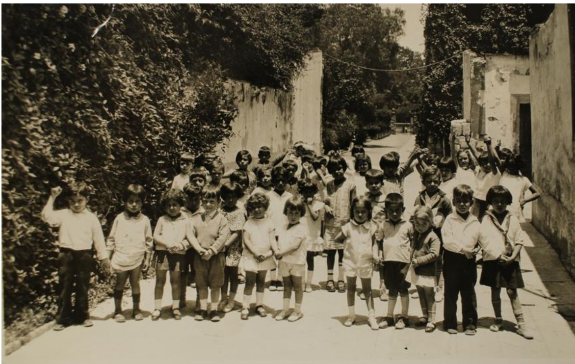
Fotografía 44: "Group of kindergartens in the driveway of their new lot. In the background is the entrance driveway and sidewalk of Colegio S. L. Keen."
