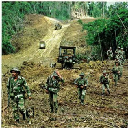
More roads mean fewer guerrillas. Or so believes the Guatemalan Army, which suffers substantial casualties while constructing new trails throughout the rain forest. Treading lightly near the Xuchil River, army road builders diligently guard against ambush and snipers.
